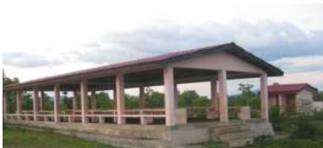
Goat droppings fill this market building in Meligo, Kailaku, because its community doesn't use it. (Image: LH)
