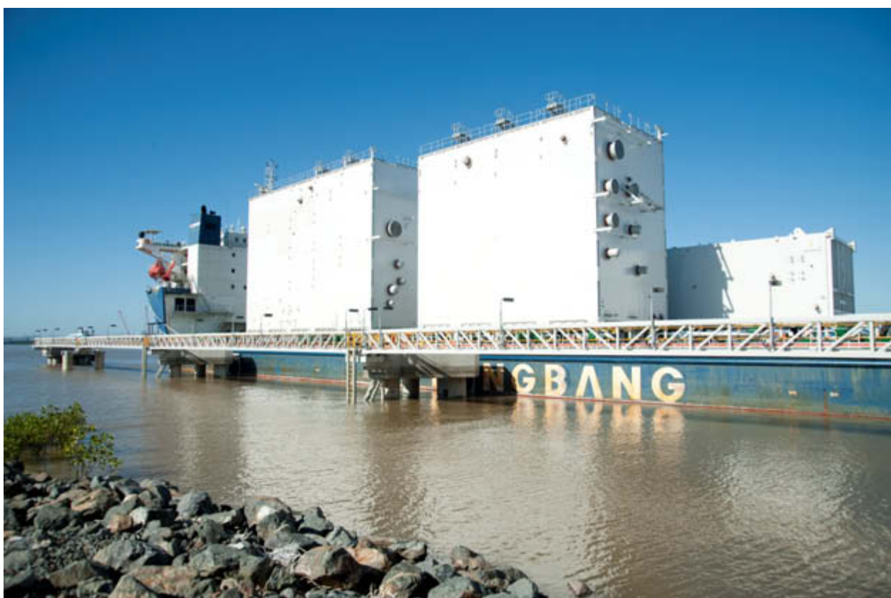
Train 1 cold boxes arriving at the material offloading facility on Curtis Island, March 2013
