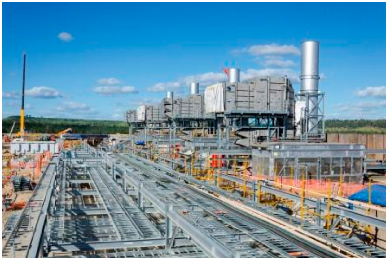
Fairview Hub-4 compressor station construction, March 2013
