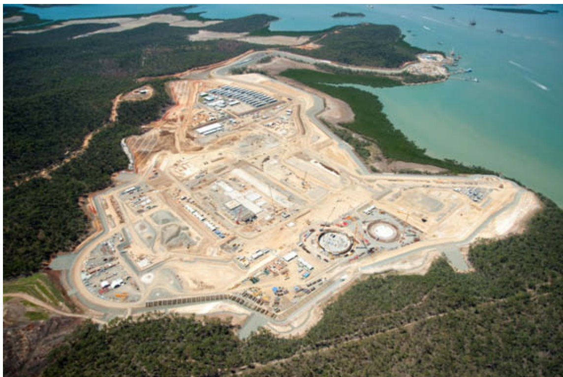
Above: GLNG plant site, October 2012.
