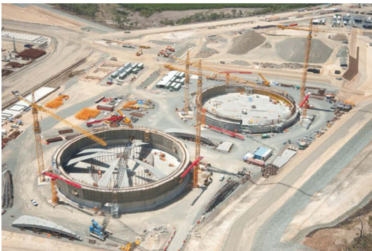
LNG tank construction, 4 January 2013
