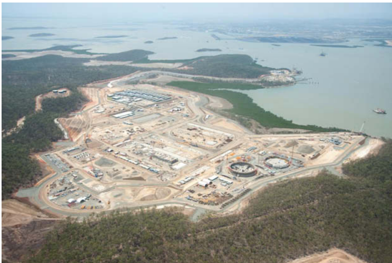
GLNG plant site, 4 January 2013.
