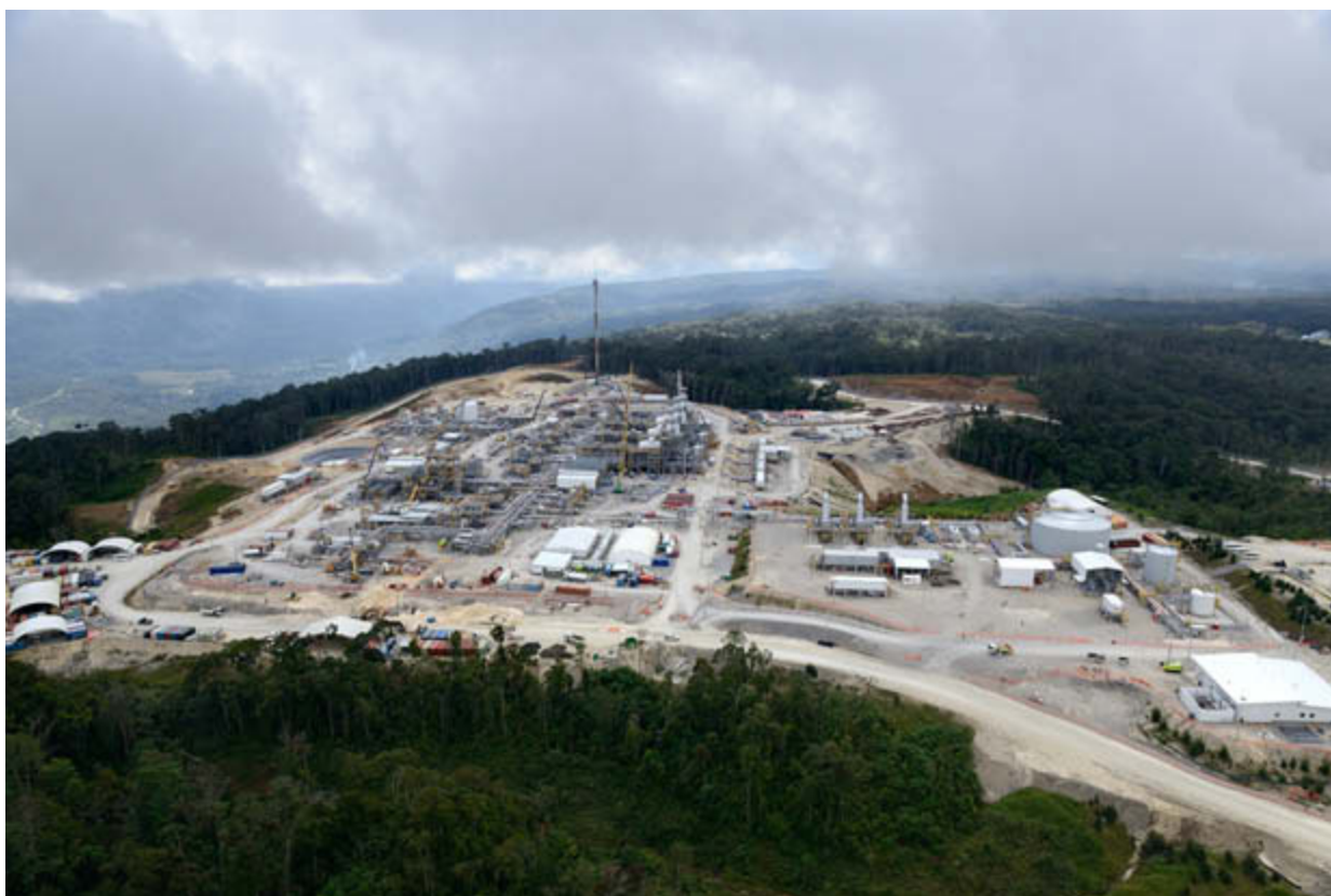
Hides Gas Conditioning Plant, PNG LNG, November 2013.
