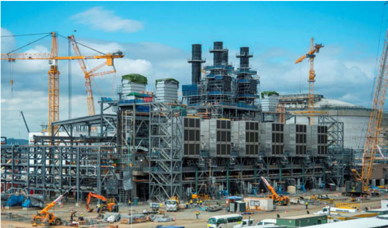
Train 1 compressor deck on Curtis Island with LNG tank B in the background, 2 December 2013.
