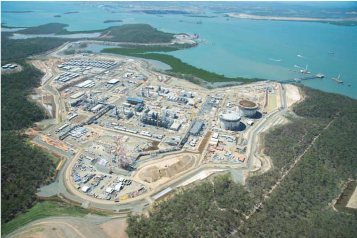
GLNG plant site on Curtis Island, 2 December 2013.
