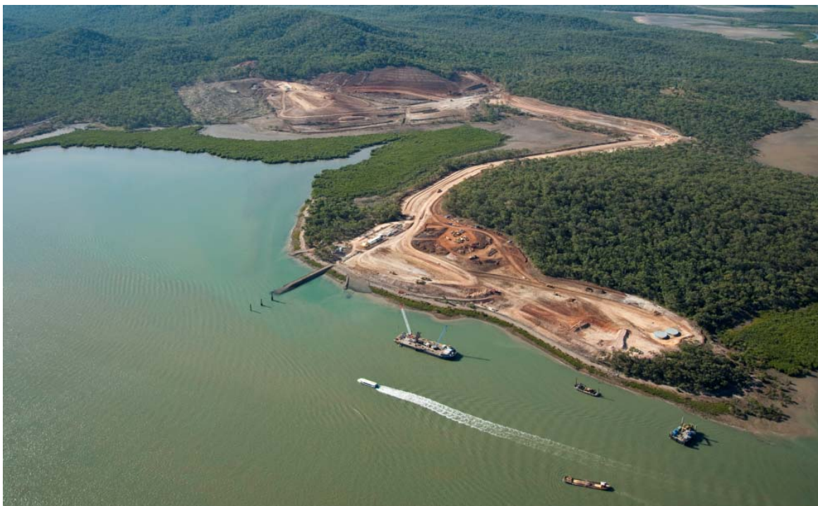
Aerial view of GLNG site on Curtis Island, 4 July 2011.
