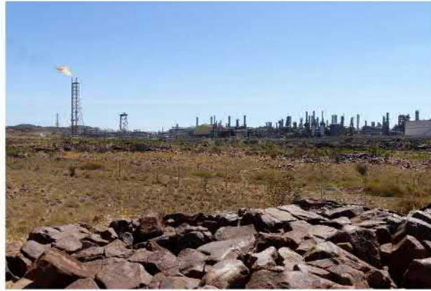
An on-shore gas processing plant in Dampier, Pilbara, Western Australia. Photo: AFP
