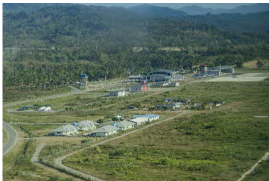
A new airport in Suai capable of receiving 200-seat jetliners was built by an Indonesian firm.
