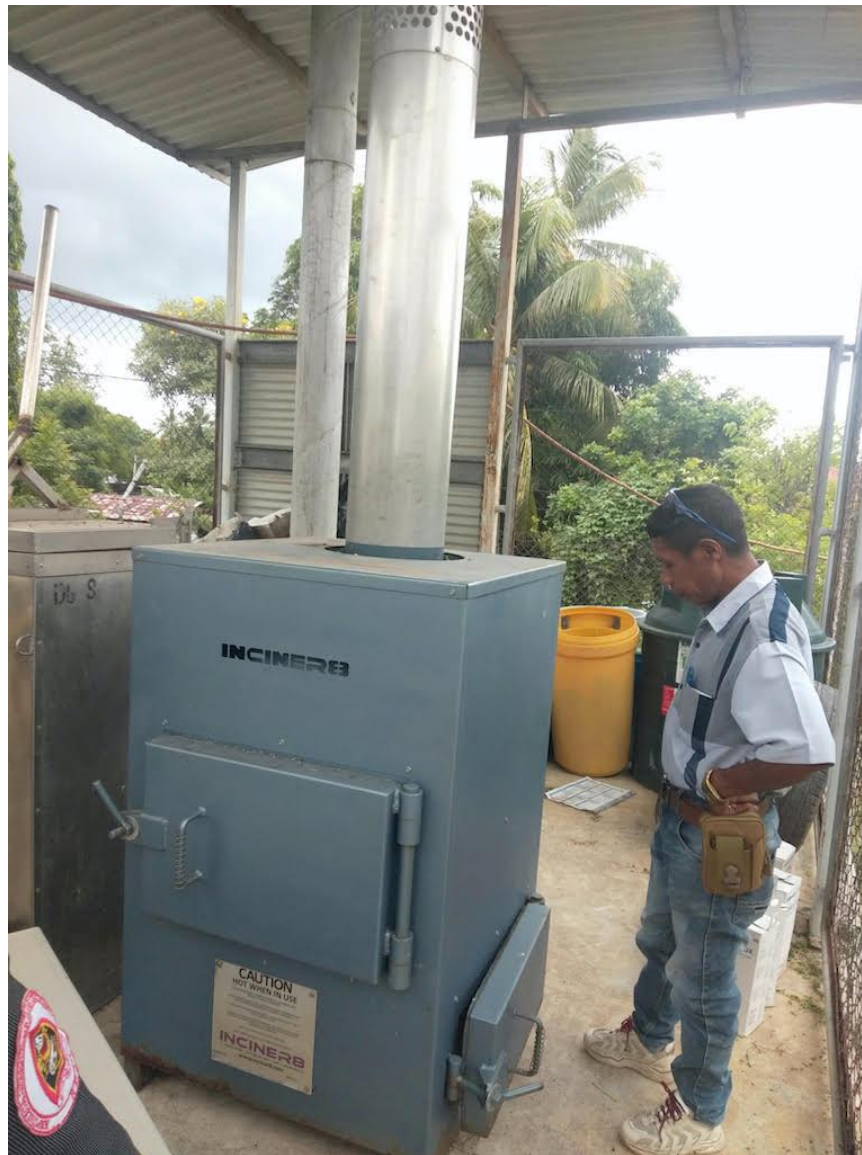
Figure 1 - Inciner8 incinerator at Suai Hospital (note: medical waste incinerator to the left not commissioned)
