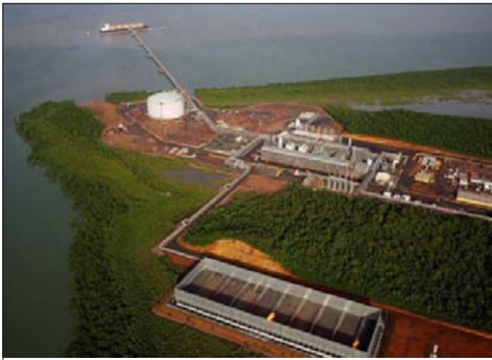
The Wickham Point LNG plant in Darwin which liquefies natural gas from Bayu-Undan. The jetty is about 1.3 km long, the storage tank is 45 m high, and the plant takes up land area equal to about 30 football fields.
