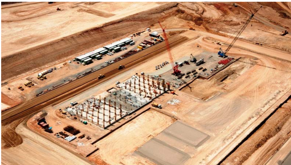
Aerial view of GLNG train-1 compressor foundations on Curtis Island, 2 April 2012.
