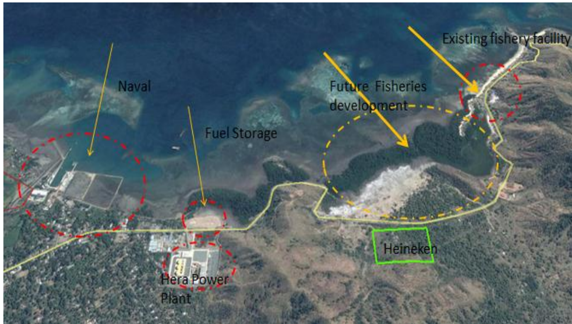
Figure. 4.22 Other Project Development in the Area
