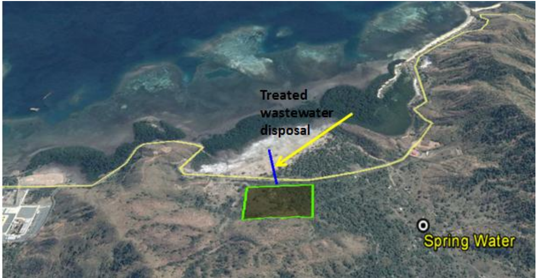
Figure 4.20 Full scale wastewater Treatment Plant and disposal to drainage ditch
