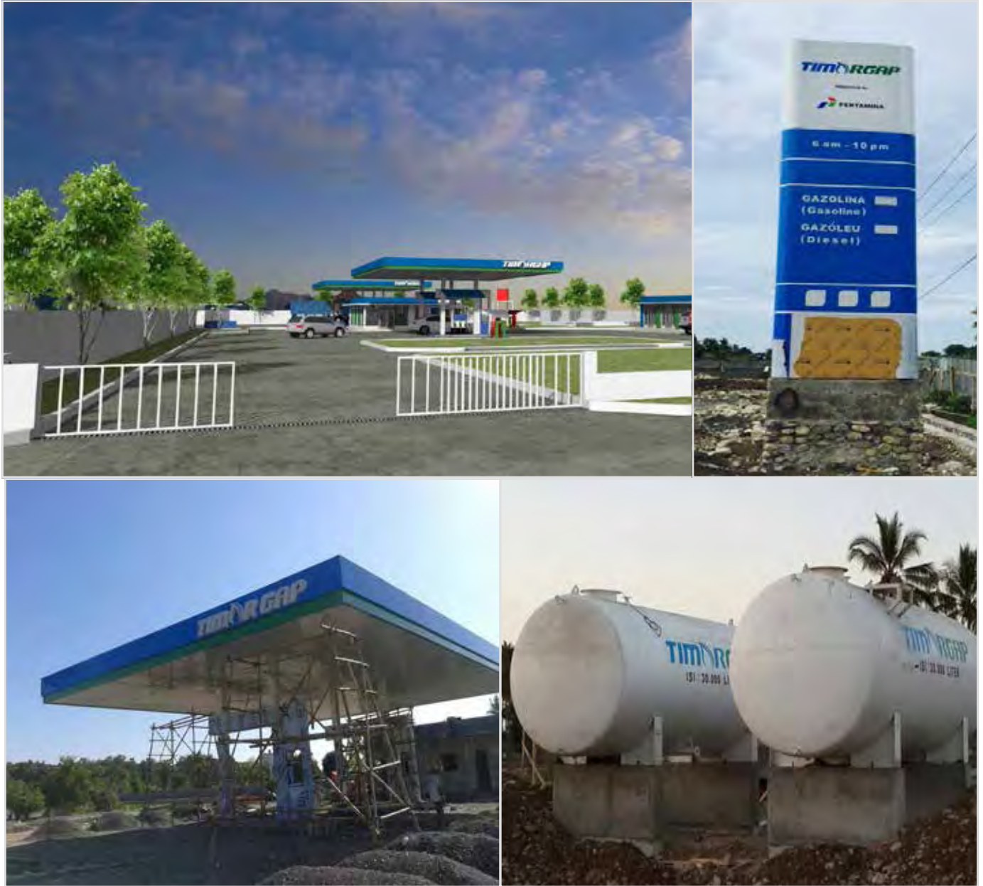
From top to bottom (left to right): Fuel station design; Fuel station and gasoil storage construction progress in Suai
