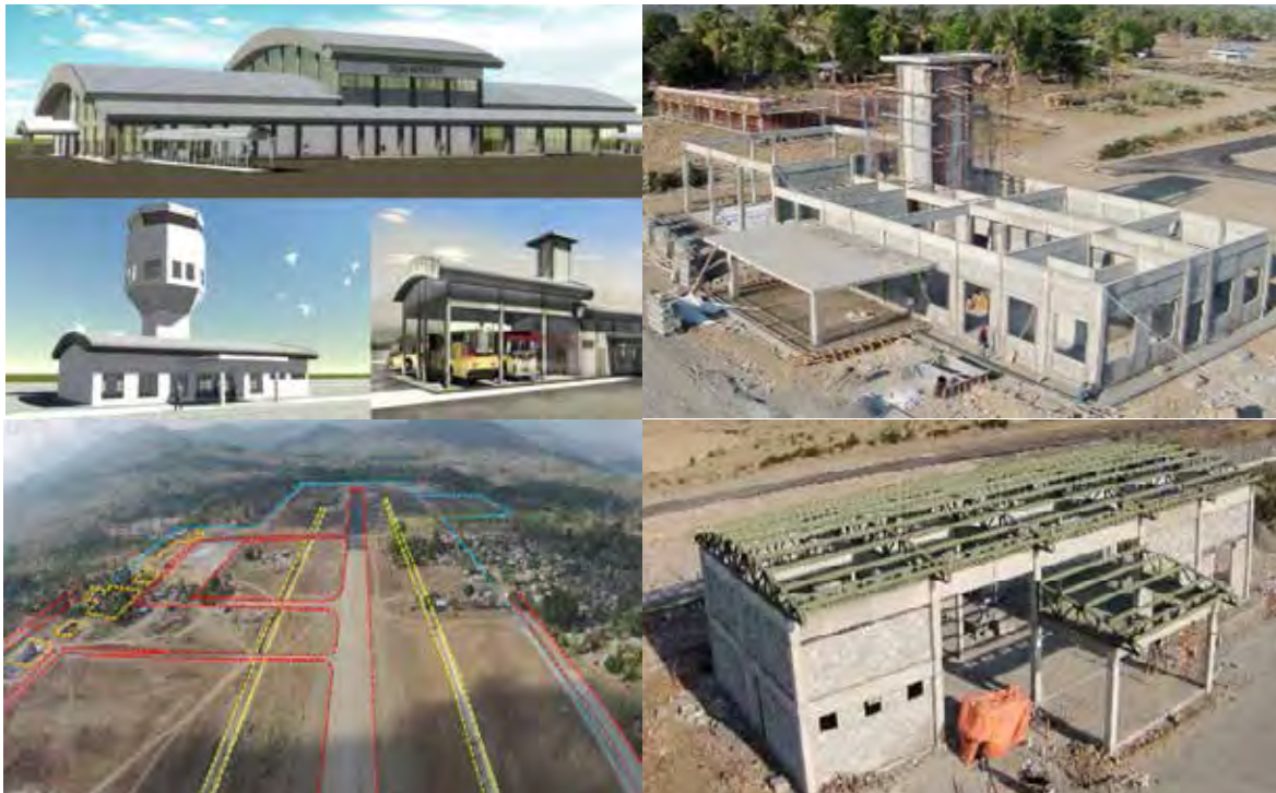
From top to bottom (left to right): Suai airport design; Suai airport construction progress; Runway total area.
