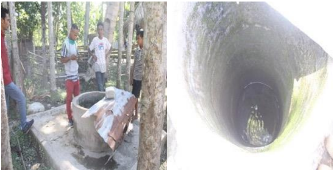
Figure 20 - Example of existing water well in Block C
