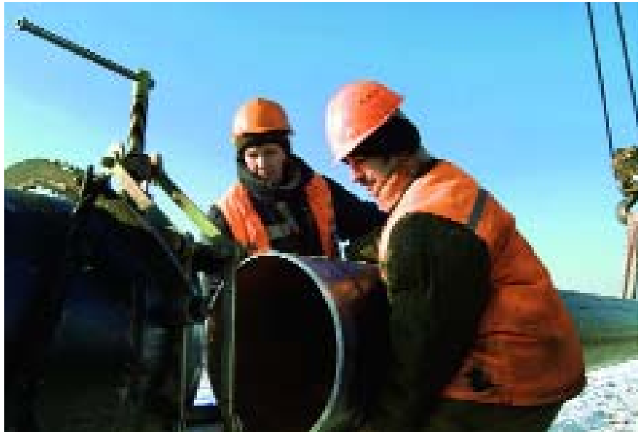
Construction of essential field infrastructure facilities, Salym, Russia
