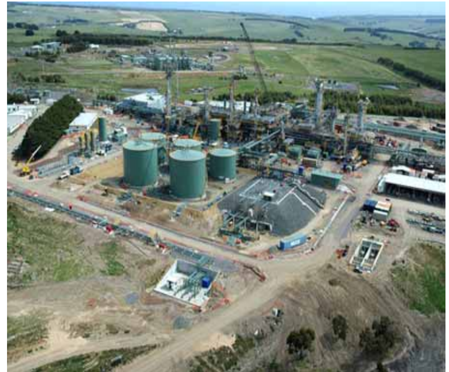
Otway Gas Plant, Port Campbell, Victoria
