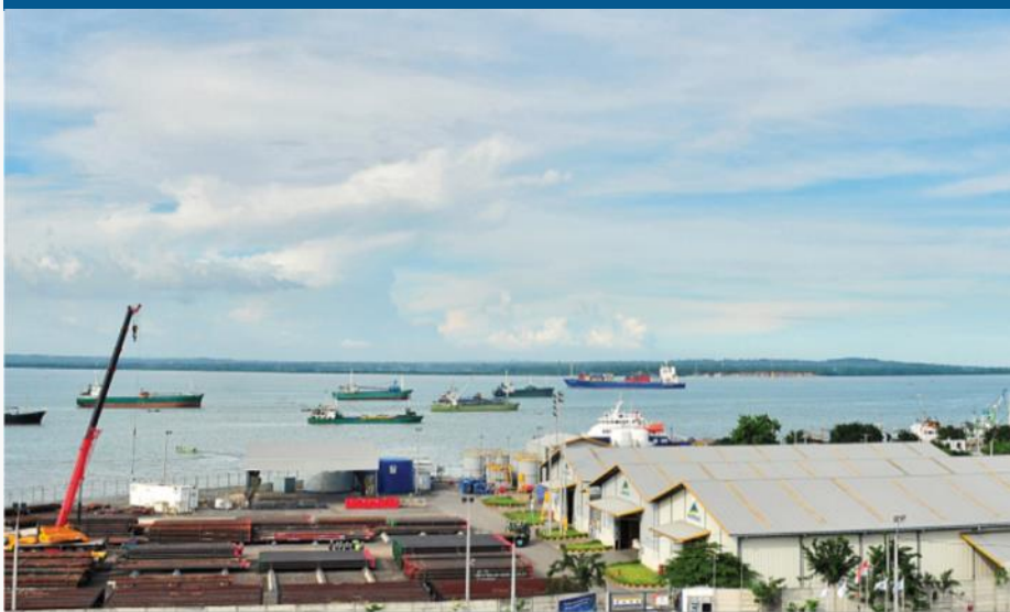
Pipe racking, fuel tanks and warehouses
