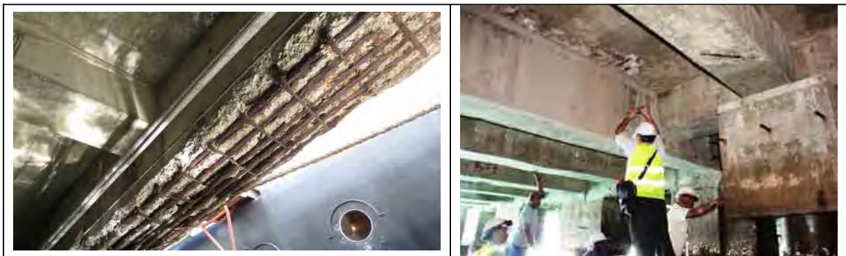
Figure 5.2-1 Inspection of Deterioration on BL5 and BL6
