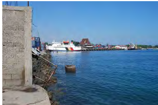
Figure 1.6-8 East Fence Seaside Edge
