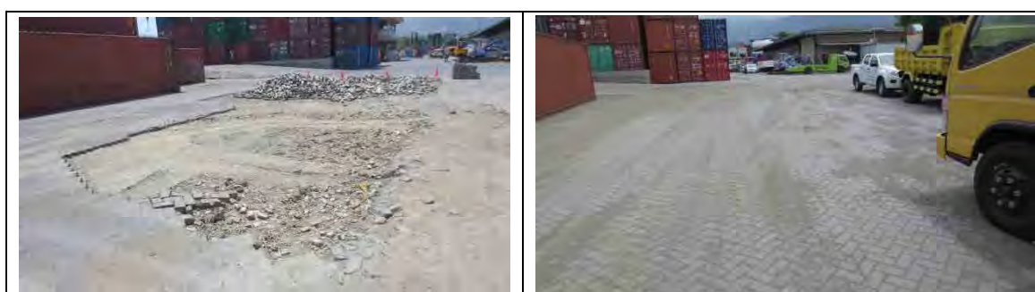
Figure 1.2-6 Improvement Area of ICB Pavement at West Side of the Yard
