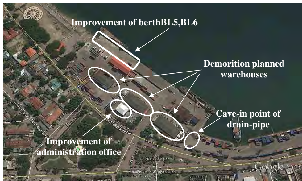
Figure 5.1-1 Facilities Requiring Repair
