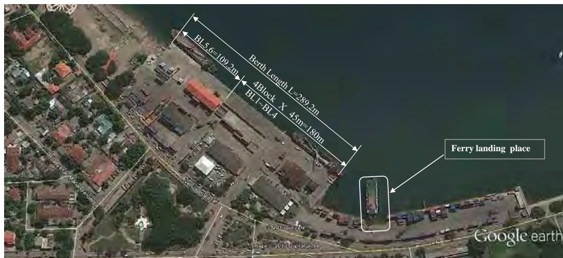
Figure 1.2-1 Mooring Facilities of Dili Port
