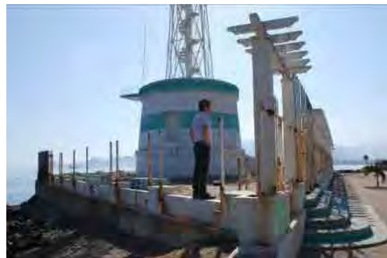
Figure 1.6-15 Fence of Lighthouse
